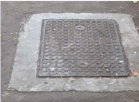
Drainage & Sewer Ducts
